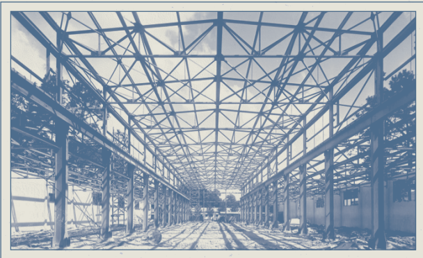
Three Sisters Warehouse, mid construction, 1941
