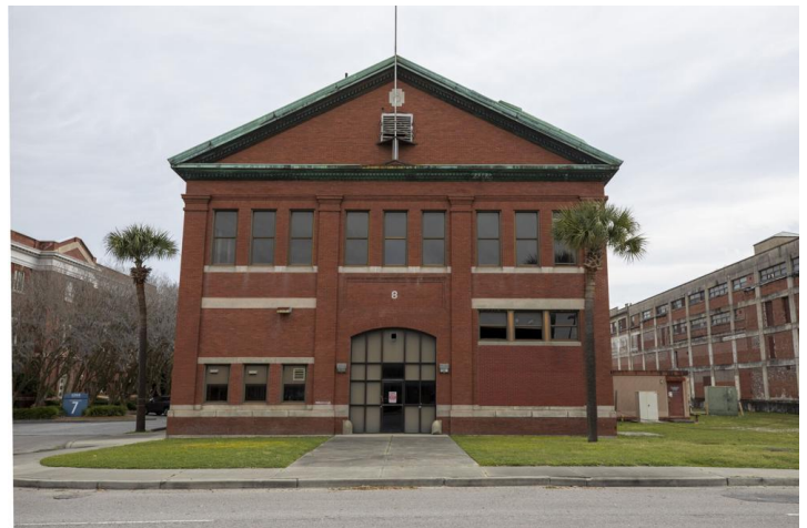
Storehouse 8 on Noisette Boulevard, on the former Charleston Naval Base in North Charleston, pictured March 19, 2021. Grace Beahm Alford/Staff
